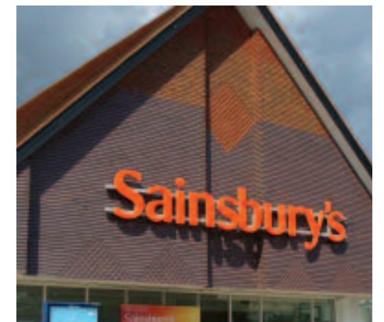
Below: The use of ornamental tiles and different colours for the vertical tiling produces a striking entrance to this supermarket.
