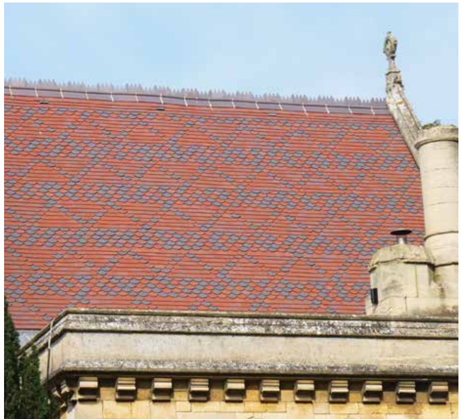
Above: Ornamental tiles in red blue blend and Staffordshire blue were used to recreate the polychromatic diaper pattern on this Gothic Revival church.
