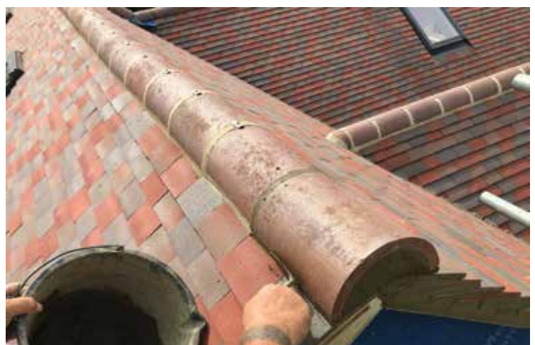
Above: A mechanically fixed mortar bedded ridge
