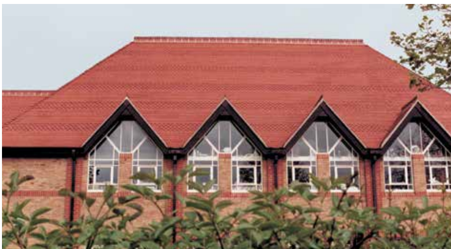
Above left: Red sandfaced tiles feature on this 2023 RIBA Small Project of the Year Award Winner by James Alder Architects. External angles, cloaked verges and monoridges were used to form a wrap over the contemporary wedge shaped extension.
