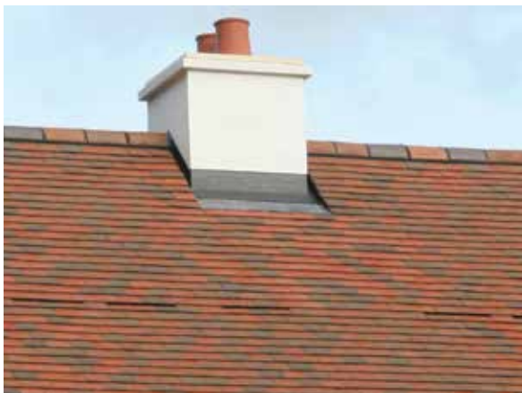
Above: Tileline tile vents providing discreet high level ventilation in the roof space
