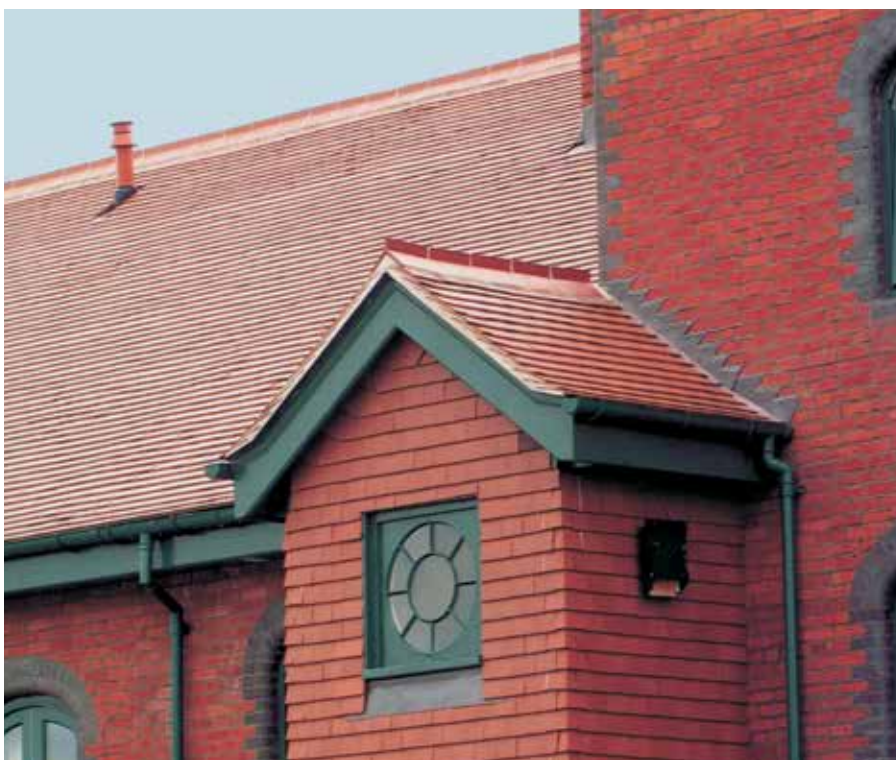
Right: Mossley Hill Hospital Liverpool Plum red tiles were used to re-roof this Nineteenth Century Hospital, special interlocking ridge tiles were made to match the originals.
