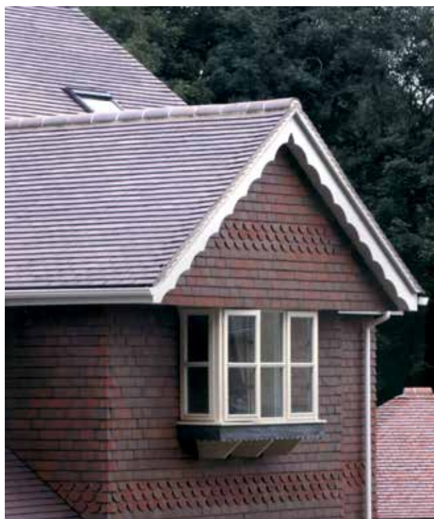
Left: On this private house, blue brindle tiles have been used on the roof, and brown antique sandfaced tiles provide contrasting shades to the vertical elevations.
