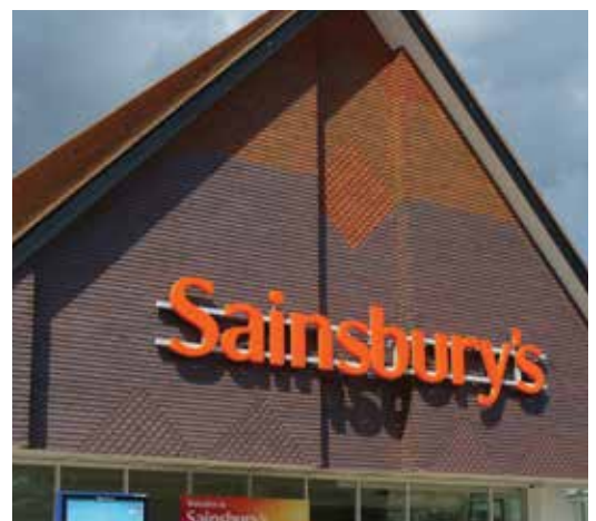
Below: The use of ornamental tiles and different colours for the vertical tiling produces a striking entrance to this supermarket.
