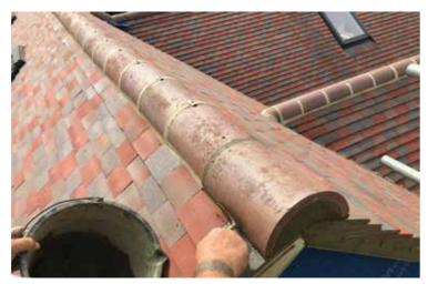
Above: A mechanically fixed mortar bedded ridge
