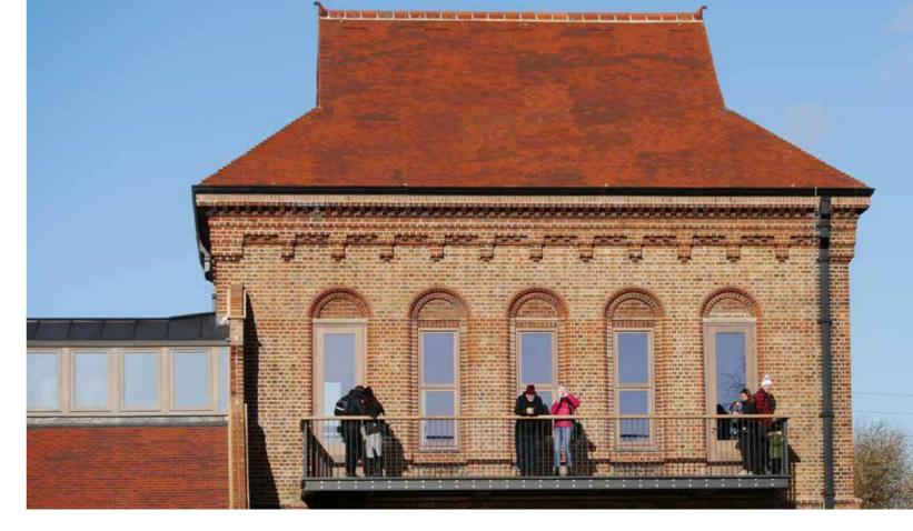
Above:Dreadnought's brown antique clay roof tiles were used to sympathetically restore the roof on the Grade II listed Engine Room at Walthamstow Wetlands in East London
