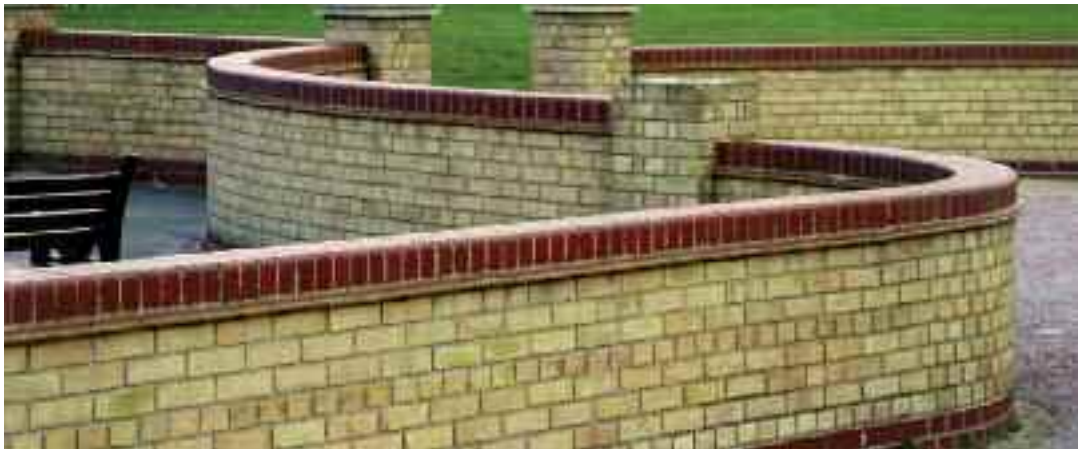
Red Double Bullnose on Red Creasing Tiles. Seafront Development, Great Yarmouth.
